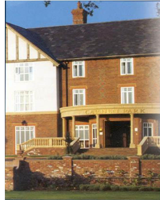
Carden Park, Chester. Recently had NICEIC Periodic Inspection carried out by Barlows (UK) Ltd.
